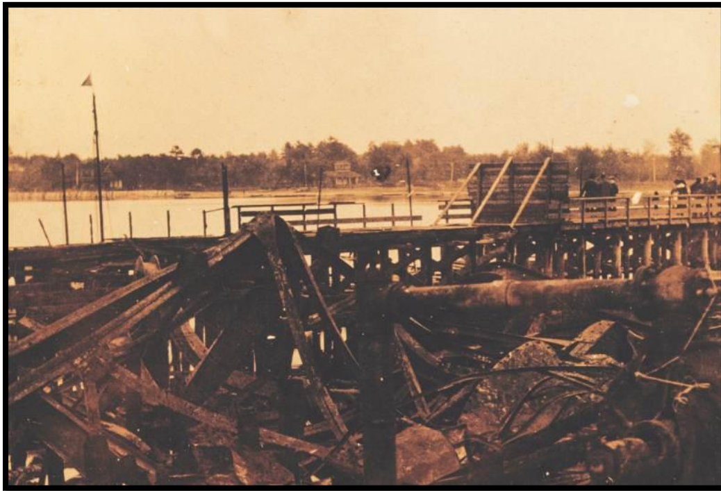
All that remains is the structural steel. Our burgee is still flying at the masthead of a boat on the other side of the pier.
